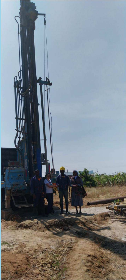
Initial work supported by Illegal Multisport Team - construction of a 300 m deep well for water extraction
