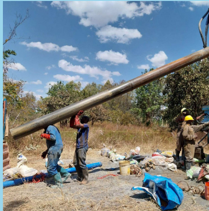
Initial work supported by Illegal Multisport Team - construction of a 300 m deep well for water extraction
